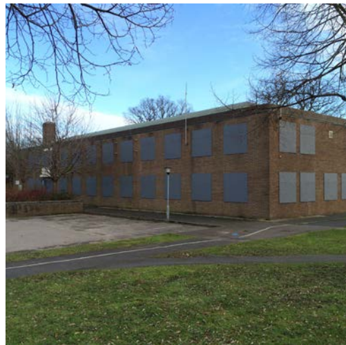
The boarded-up Police Station building
