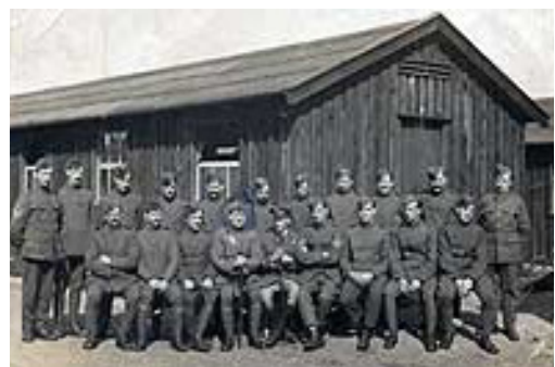
The Pinehurst Barracks (Elles Barracks from 1934) which was demolished in 1970s. The Sergeants Mess is used as the Farnborough Community Centre
